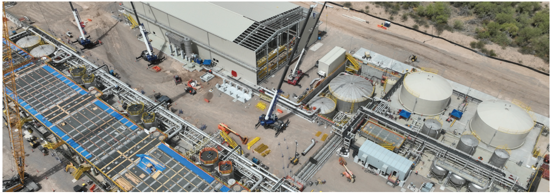
Florence Copper construction site, March 2025
