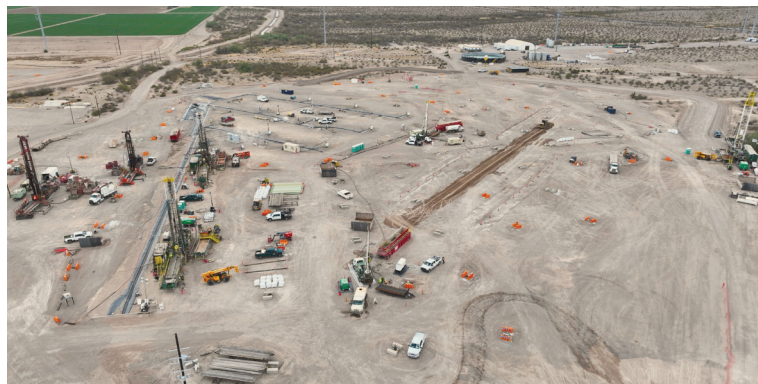
Florence Copper wellfield construction site, February
